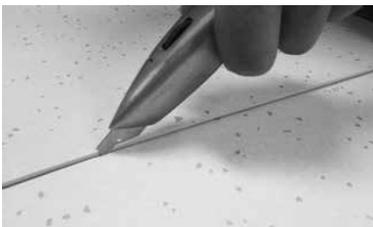
Finish cutting the seam using a utility knife with a hook blade to provide a slight undercut (image 4). Do not damage the Eclipse-GF 020. Carefully remove the excess material.
