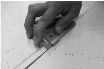
If the seam is not going to be welded or if the factory edge is damaged, use a Crain 340 selvage trimmer or similar to trim off ~0.5 inches (image 1).
