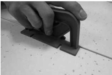
Next, or for welded seams, use a knife with the blade set at just under the thickness of the flooring, carefully trace cut the entire seam (images 2 and 3). A utility knife (used vertically) with the same type of straight blade is needed to finish the cut at each end.
