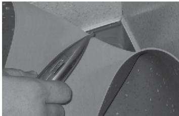
Dry-lay the flooring as detailed above and make relief cuts at all corners to avoid any rips. Push the flooring into the internal corner as far as possible without damaging the flooring. Cut a straight line starting at the base of the cove stick up through to the top edge of the flooring at approximately a 45° angle (middle) (image 1). Do not trim the perimeter or internal corners until the field flooring is adhered.
