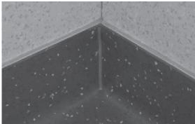
For all internal corners, place one side into position and trim off the excess material, resulting in a straight cut down the center of the corner and through to the base of the Staticworx cove stick. Repeat the process with the second side. A slight gap is acceptable as all internal seams should be cold welded (image 3).
