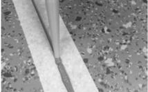
Inject the cold weld into the groove without gaps until a small bulb develops above the seam (about the size of heat weld rod) (image 1). At the end of the seam, release the gun to prevent leaks. Any cold weld tracked or spilled on the flooring must be removed immediately using 70% Isopropyl alcohol or liquid soap and a clean cloth, as cleaning at a later stage may not be possible.
