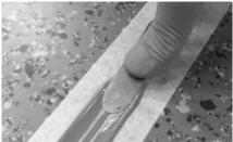
Press the cold weld into the seam using a smoothing spatula, held nearly flat (~22° angle), resulting in a surface flush and on the same plane as the surface of the tape (image 2). Excess cold weld must be pressed away on each side of the seam. It is important to develop a slight gap between the excess weld and the weld within the seam for easy removal.
