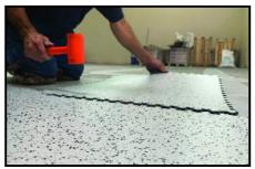
Proper flooring is a necessary part of any ESD control program.
