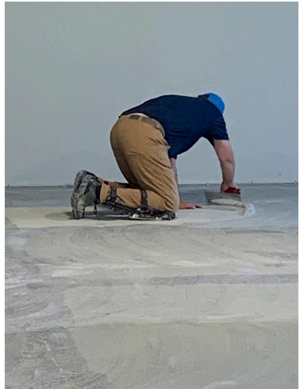
Figure 2: Adhesive installation
