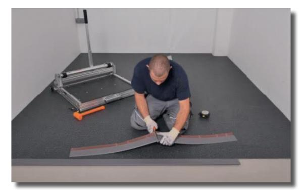
GLUE: Remove protective film from adhesive tape
