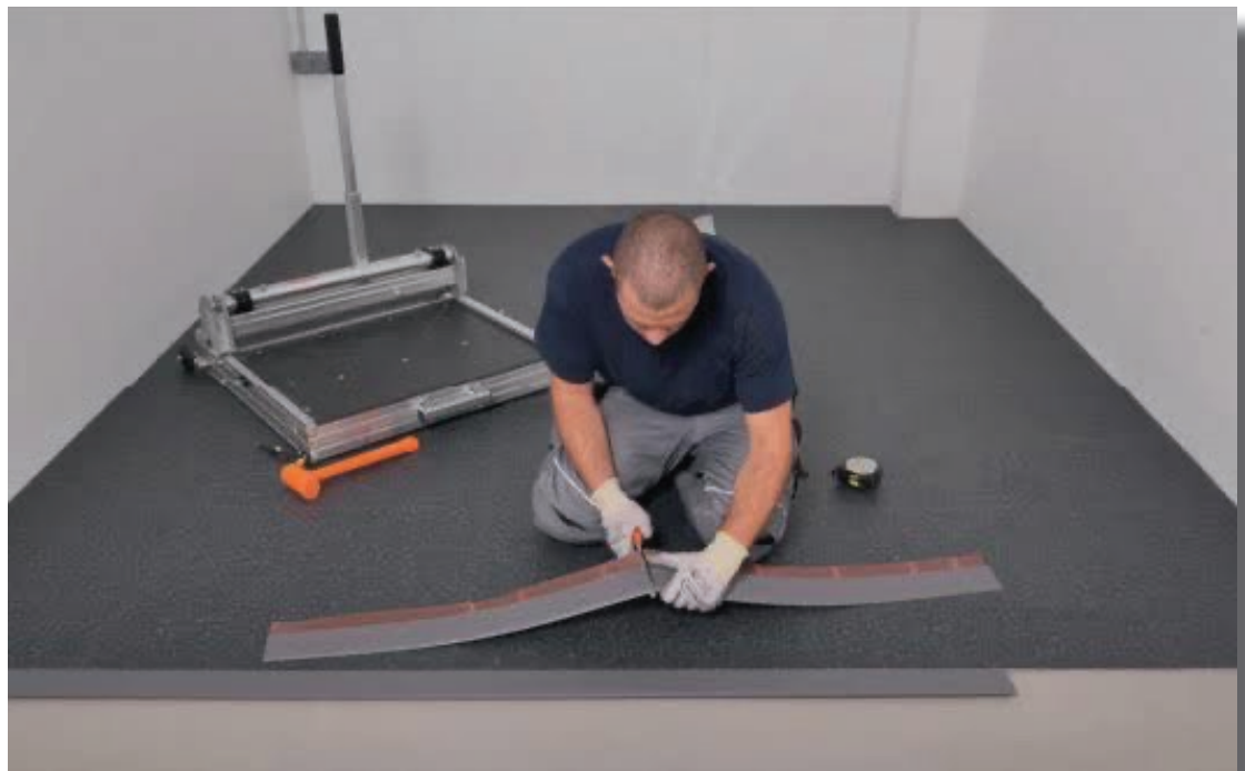
GLUE: Remove protective film from adhesive tape
