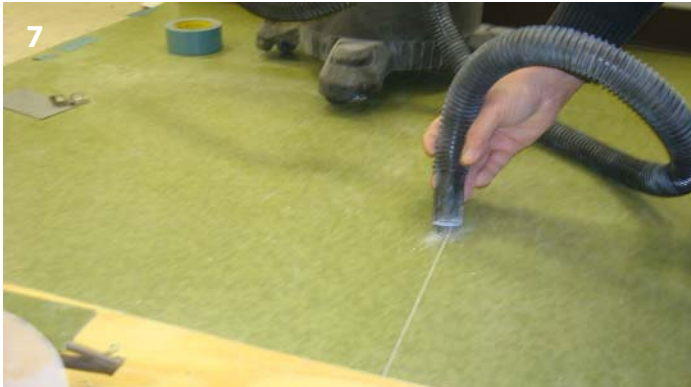
Vacuum all seams to eliminate welding problems and open seams.
