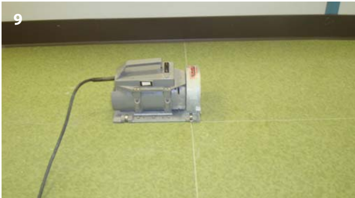
Router all field seams in one direction only, being careful to keep the groove centered on the seam as closely as possible. Using chamfering plane to router cove pieces where the route cannot be operated.
