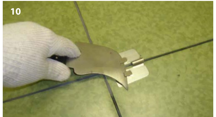
Removing the excess bead from one direction before working the bead from the opposite direction.
