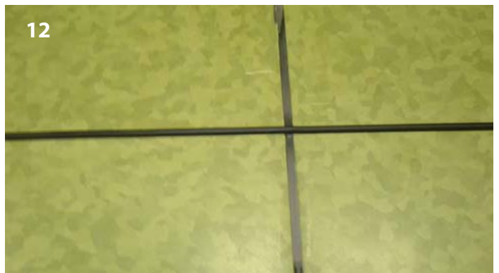
A lower heat is recommended for correcting mistakes or welding in awkward places. A good weld is achieved when a small amount of melted bead overflows along the edges of the groove.
