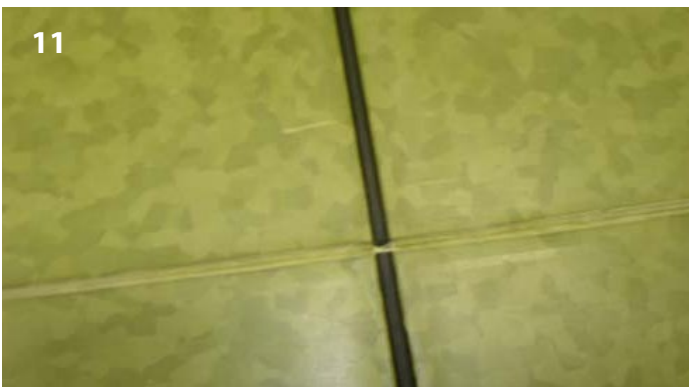
Angle cut or router your bead at the junctions to make it easier to weld in the opposite direction
