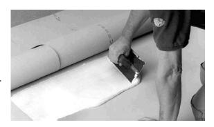
have a milky appearance. Dry time will depend on subfloor porosity, ambient temperature and humidity. Apply flooring within a maximum of 4 hours after the adhesive has dried to the touch.
